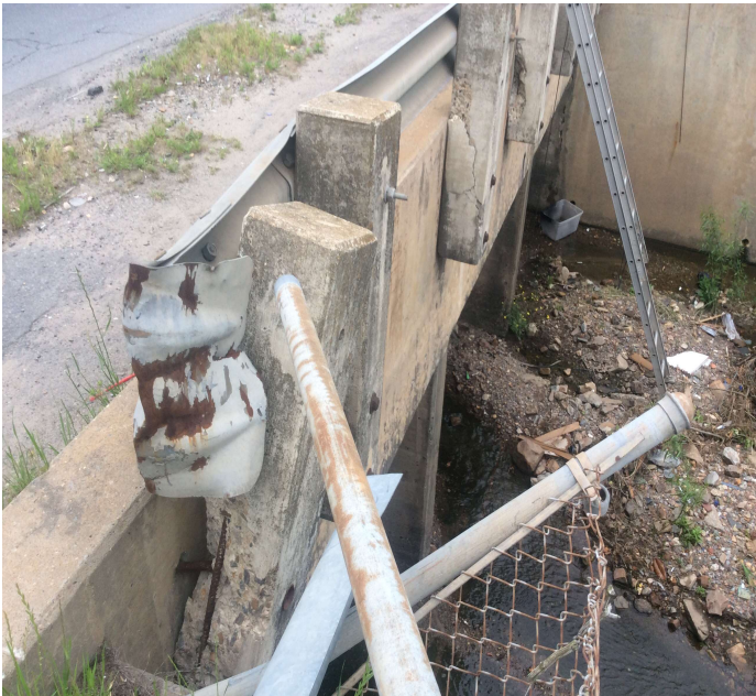
PHOTO 1 Description Right bridge rail damaged due to traffic impact.
